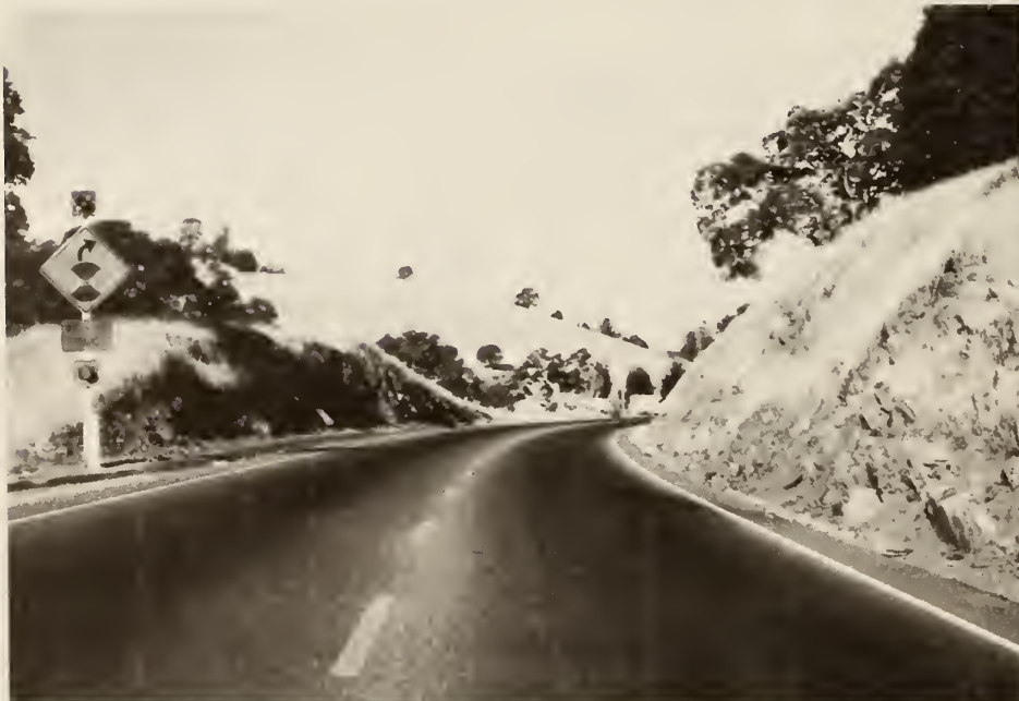
Figure 60 Activated Advance Warning Device (Amador Central Crossing)
